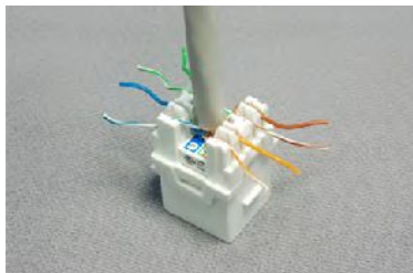
2. Place the wires into the slots according to the wire scheme.
